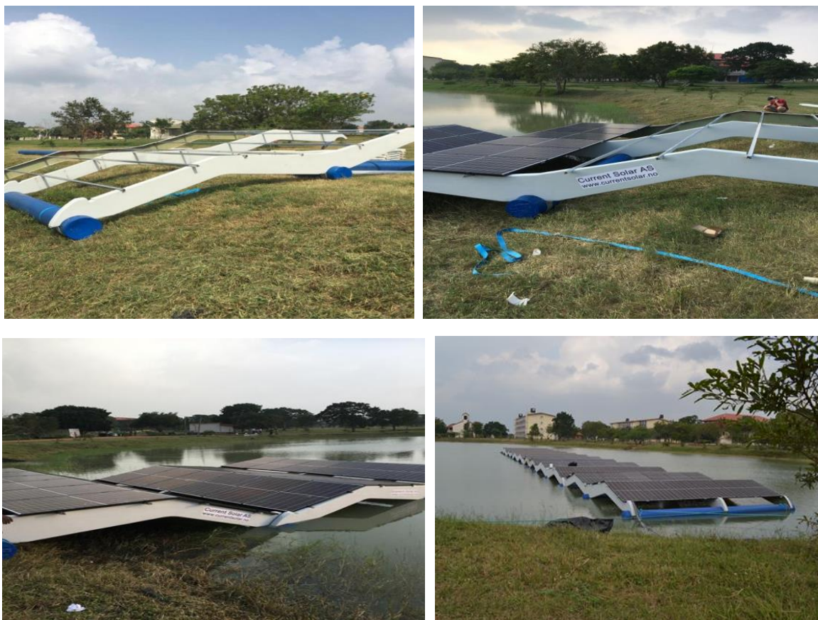
Figure 2: Floating solar plant Installation step by step
